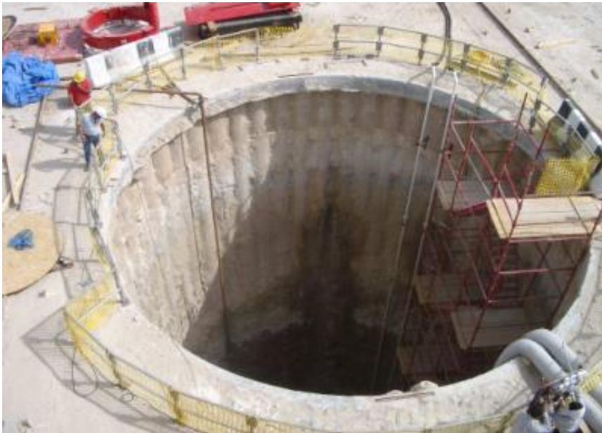
Figure 5.1: Shaft being Constructed by Secant Piling Method
